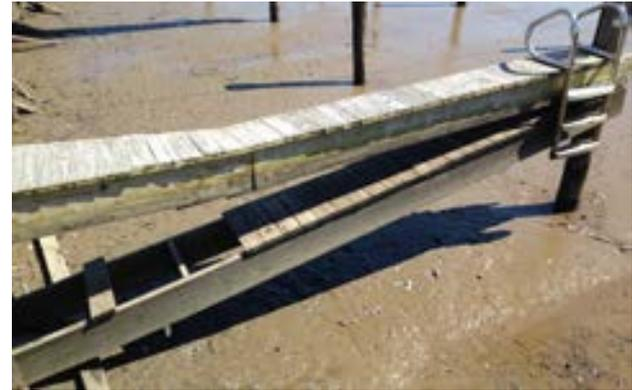
*A finger pier that is rotten and collapsing, 2014*
